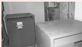
These service structures are located inside a building "closet" so that the structures are incorporated into the development and not visible from adjacent properties. The "closet" is accessible from the exterior ground level.
