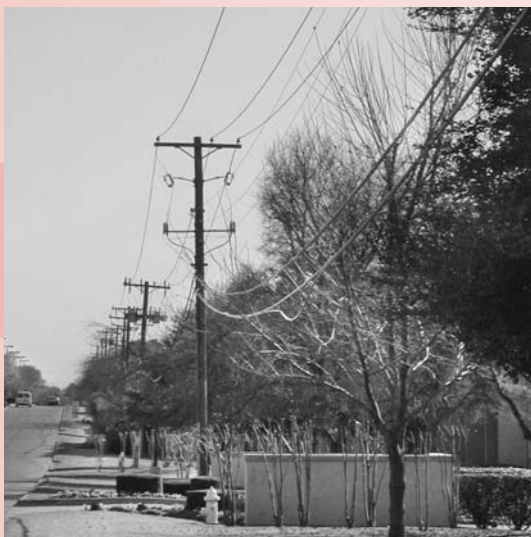
Overhead infrastructure is visual clutter that detracts from the aesthetics of a community, such as along Marsh Lane in Farmers Branch
